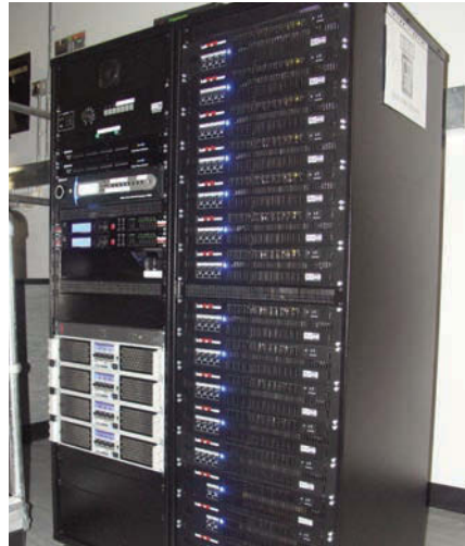
◀ A clinically clean projection room (far left), is host to the latest projection and audio kit including a 56-channel Dolby Atmos installation (left)
