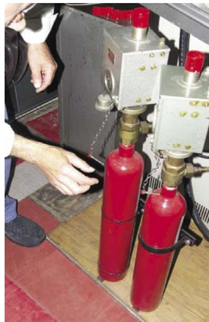
*Withdrawing pins - activating CO2 plungers*
